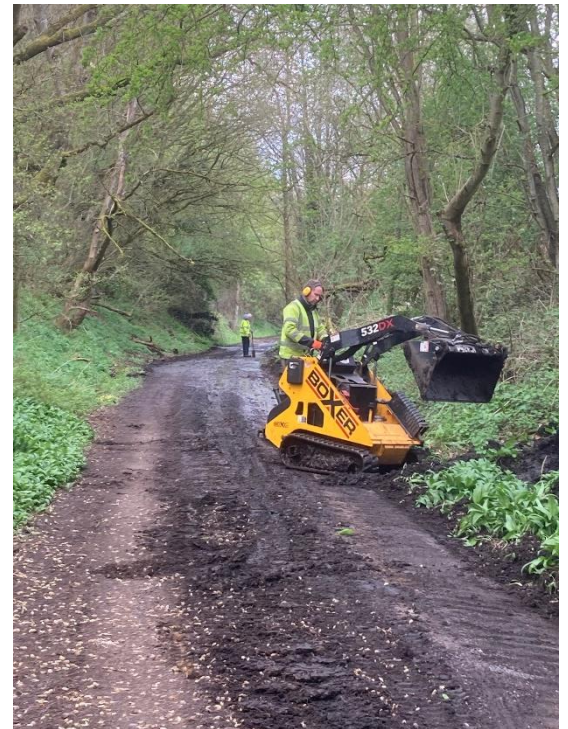
Mud-scraping on the disused railway line near Black Dog Halt.
